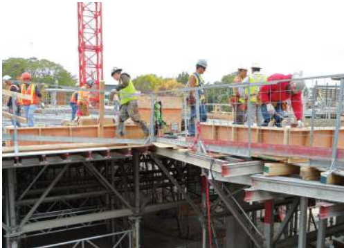
Construction Site and Temporary Office
